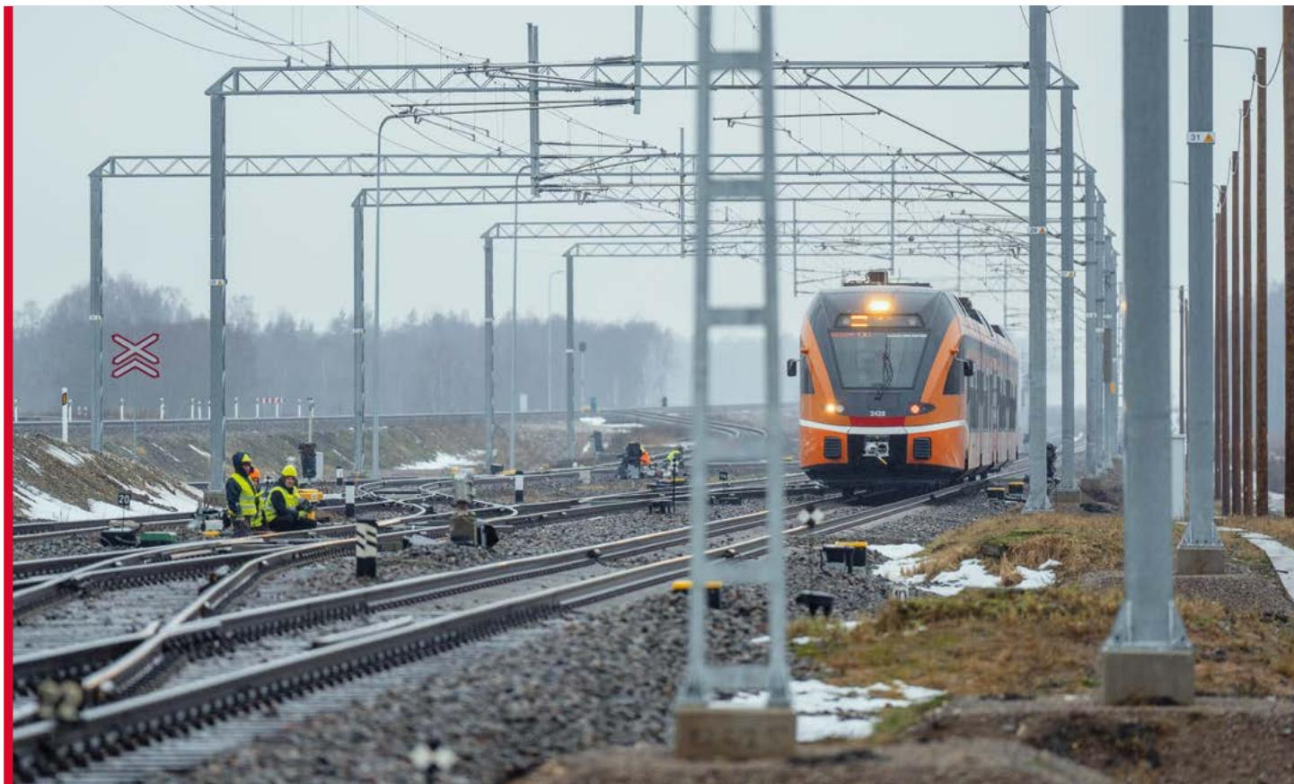
**Straightening Curves and Major Overhaul of the Tartu–Valga Railway Line.** The work involves straightening the Palupere–Puka sections (10.2 km) and a major overhaul of the Puka–Keeni section (11.4 km), the removal of the Puka station, and the construction of 7 culverts. The majority of the work will take place between 2026 and 2027.
